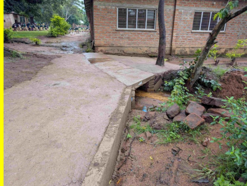
Water bridge completed forming a corner intersection walkway.
