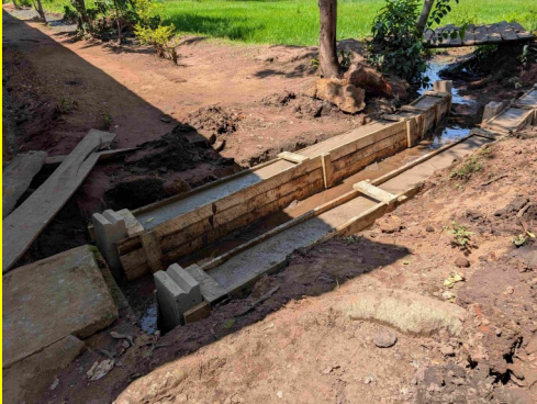
First stage of construction consisted of a small water bridge.
