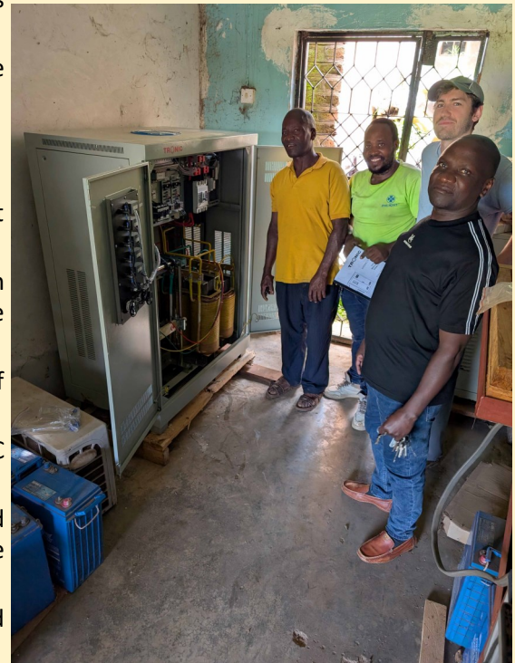
Fodias, Barton, Nathan and Menard standing beside the new hospital stabilizer.
