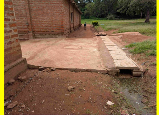
Culvert added to channel water and provide an entrance driveway.
