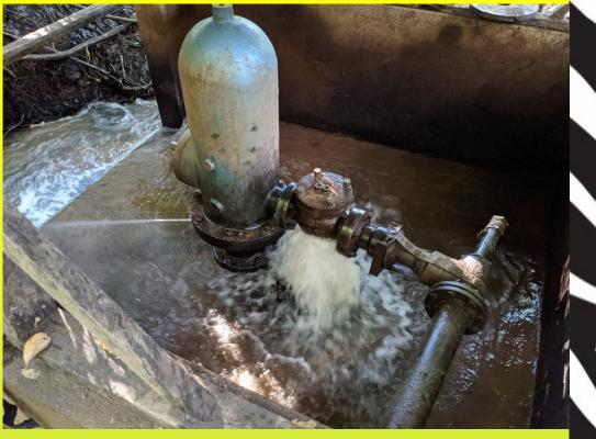
canal) to a holding tank at a higher elevation. This water is then stored and then deposited all over the mission, from outdoor spigots to the hospital water purification tanks, with zero electricity. In the 1980s, the hydram was replaced, and further work and maintenance was done on that model for the next four decades.
