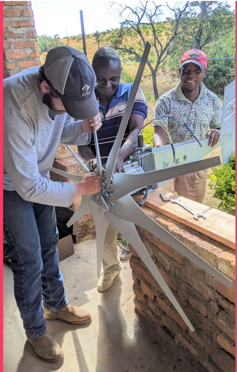
Nathan, John "Sparky", and Naaman working on the wind turbine at the Ailsa farm house.
