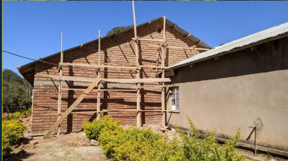
Foundation and floor plan in the beginning stages of construction.
