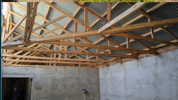
Inside walls are plastered, with wood rafters and roof sheets visible.
