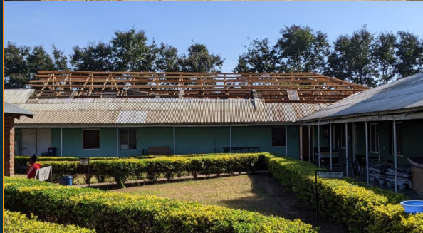
Inside hospital view shows joining of new construction with existing structures.
