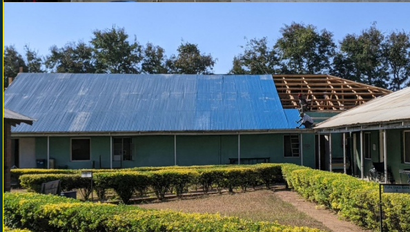
New roof sheets give surgical theater a uniform appearance.
