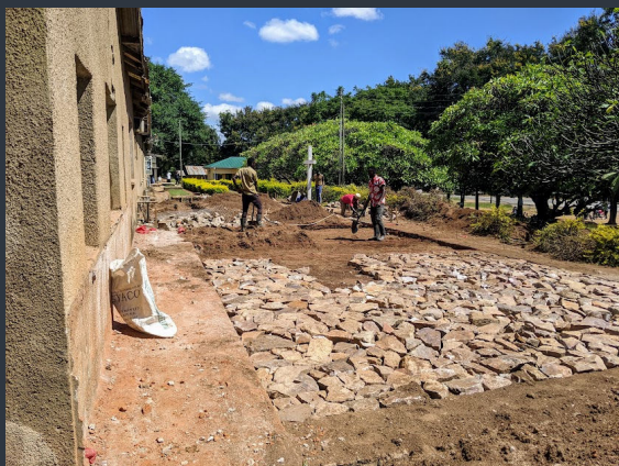
Workers laying the foundation of new operation theater addition.
